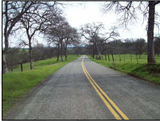
Platina Road – Typical area where disc trail fuelbreaks could be constructed
